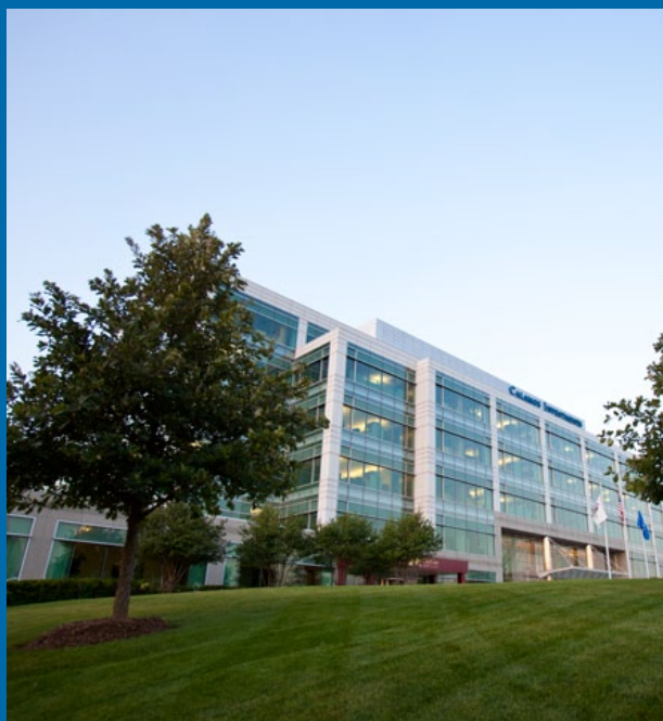
Calamos Global Headquarters Naperville (Chicago region), Illinois, USA
